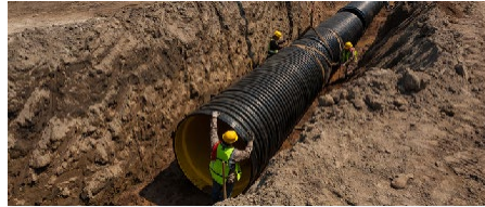
Localized Flood Mitigation Projects
